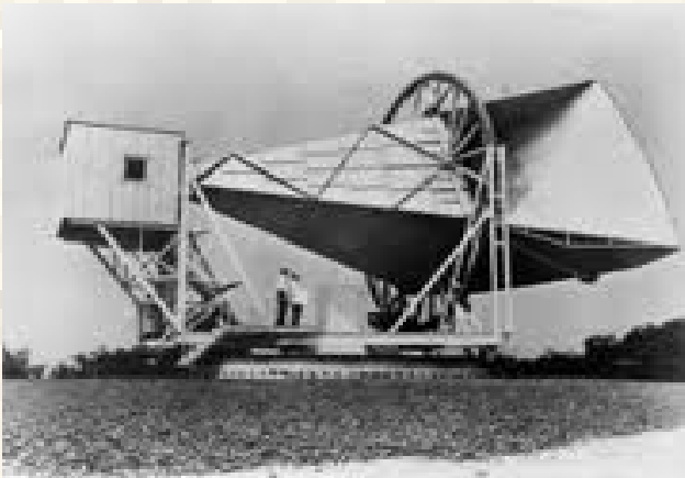
Holmdell horn antenna, 15m length 4.08 GHz
